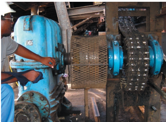
Sugar cane processing equipment with Cooper bearings in trapped positions.
